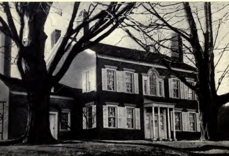
NOBLE HOUSE, NEW MILFORD
